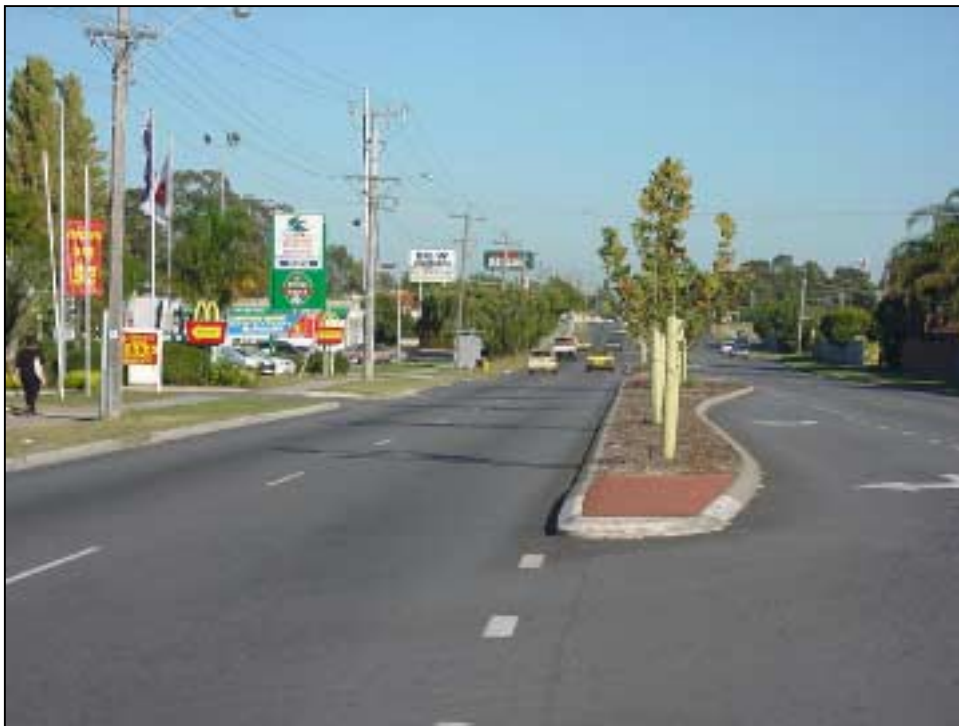
Figure 1 View of High Road from Cerberus Ave. (Estimated 30yr traffic of 2.6 \times 10^6 ESAs)
