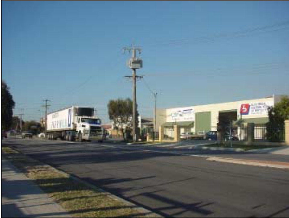
Figure 3 View of John Street from Charles Street (Estimated 30yr design traffic 5.1 \times 10^6 ESAs).
