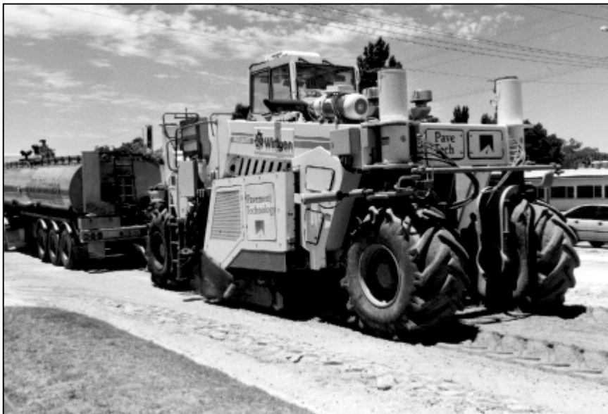
Figure 4 The Wirtgen 2500 reclaimer/stabiliser was used for stages 1 and 2.
