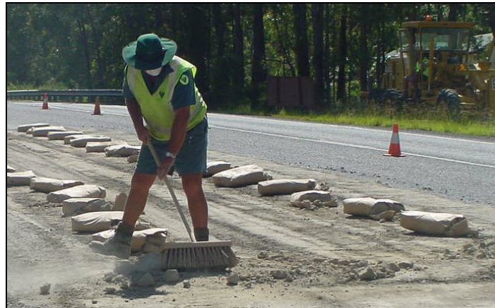
Figure 2 Better uniformity is likely to be achieved with raking or brooming on a firm rather than loose surface.
