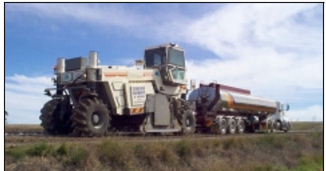
Figure 1 Foamed bitumen insitu stabilisation using a modified specialist reclaimer.
