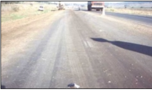
Figure 4 The hard surface of the road after foamed bitumen stabilisation.
