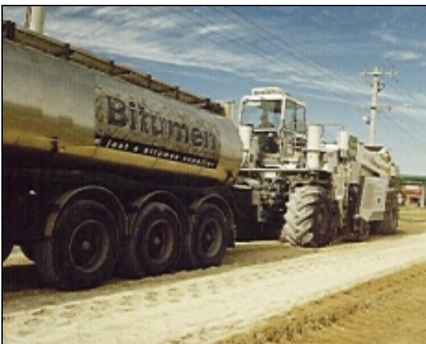
Figure 7 Tanker coupled to reclaimer during stabilisation stage.
