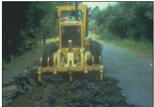
Figure 2 Tying an existing road with a grader attachment.
