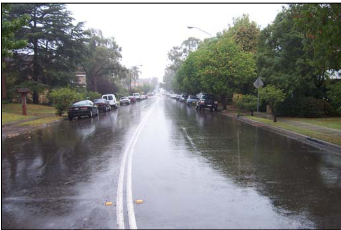
Typical local road in Sydney with foamed bitumen stabilised base.
