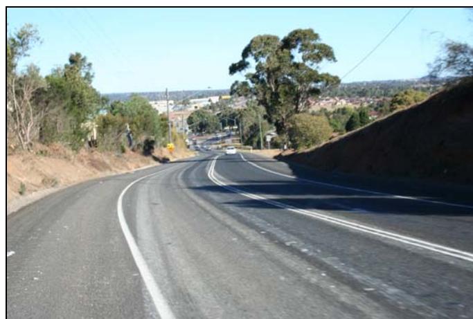
Campbelltown Road after stabilisation and prior to the asphalt base layer.
