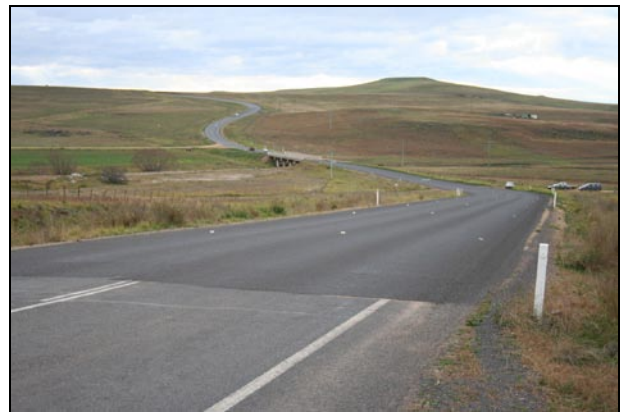
Stabilisation with Polyroad for rehabilitation of the Monaro Highway at Rock Flat Creek, just south of Cooma (NSW).
