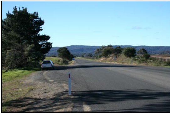
Foamed bitumen stabilisation used for rehabilitation of the Princes Highway at Quaama (NSW).
