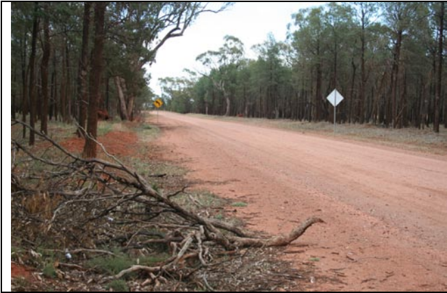
Willow Road, Coolamon (NSW) was lime stabilised in 2001 at a depth of 150 mm with 3% design lime application rate.
