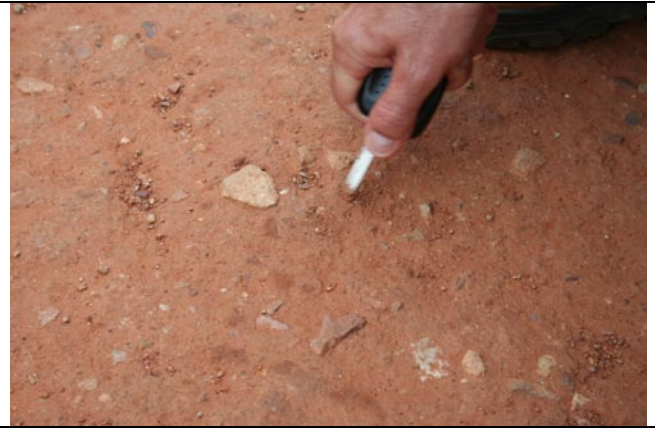
Willow Road, Coolamon (NSW) was lime stabilised in 2001 at a depth of 150 mm with 3% design lime application rate.
