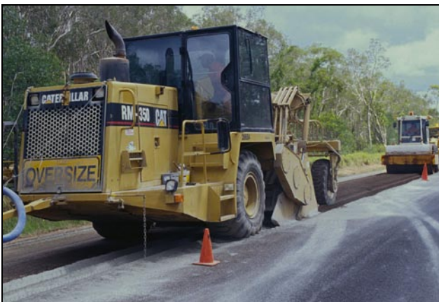
One of RoadTek's CAT RM-350 in operation in western Queensland.
