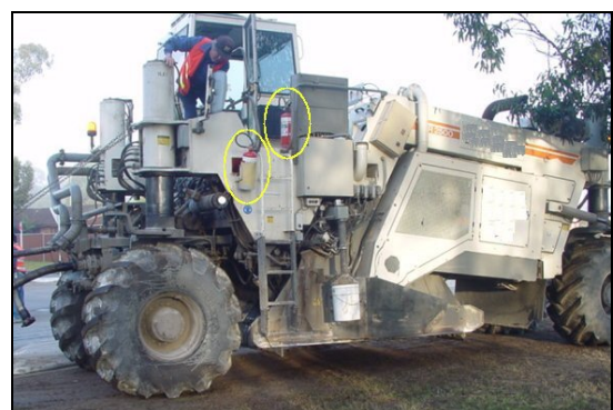
Figure 4. View of two 9 kg fire extinguisher on reclaimer.
