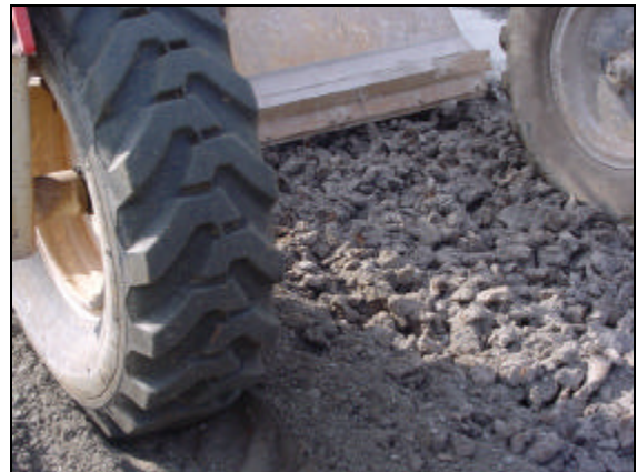
Figure 4 The first mixing pass with heavy clays will produce material with large pieces of clay.
