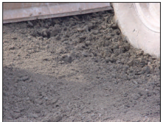
Figure 5 Subsequent mixing passes with heavy clays will produce finer material suitable for compaction.
