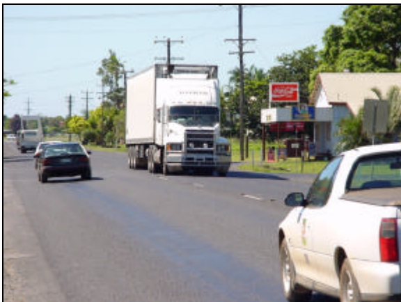
Figure 7 Foamed bitumen stabilisation as base course material for Bruce Highway Innisfail, Queensland.
