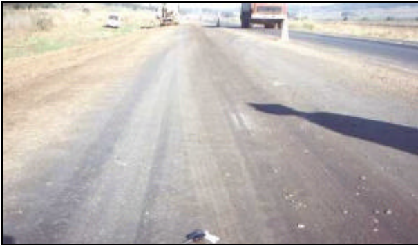
Figure 4 The hard surface of the road after foamed bitumen stabilisation.
