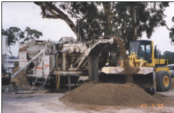
Figure 2 Foamed bitumen stabilisation using a mobile batch plant. The material is placed using conventional road making and/or asphalt laying equipment.
