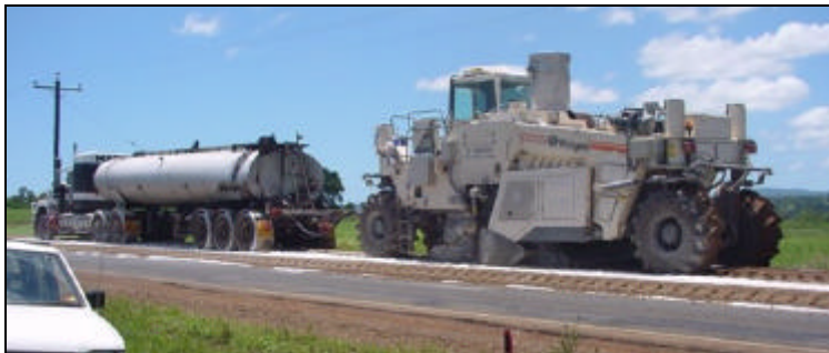
Figure 1 Foamed bitumen insitu stabilisation using a modified specialist reclaimer.
