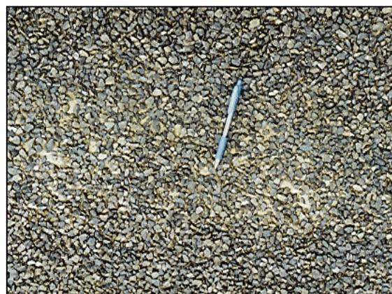
**Figure 5** View of stabilised pavement with 7 mm crushed aggregate on surface.
