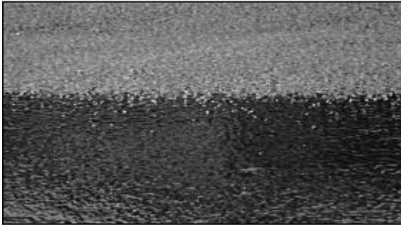
**Figure 6** *View of stabilised pavement with seal and 7 mm crushed aggregate as a wearing surface.*
