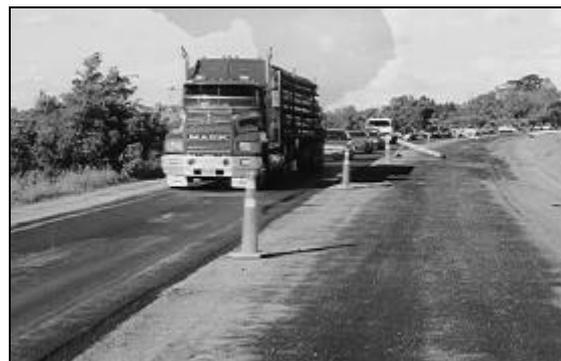
**Figure 4** A stabilised pavement with a cementitious binder undergoing moist curing and open to heavy traffic.
