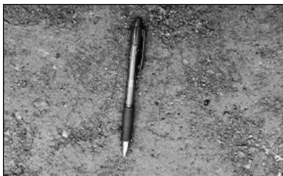
**Figure 3** Fine micro-cracks develop on the surface in a stabilised layer, but pose no detrimental problems.
