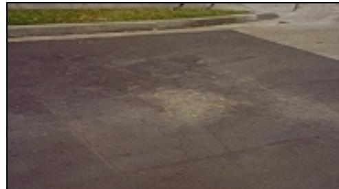
Figure 1 This patch did not resolve the underlying subgrade strength deficiencies.
