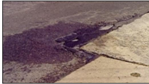
*Figure 3 The presence of localised surface water indicates that there is a problem with drainage of the pavement material.*
