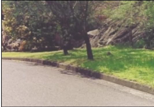
*Figure 2 The closeness of the rock adjacent to the footpath indicates that rock is close to the surface or rock floaters may be near the surface.*
