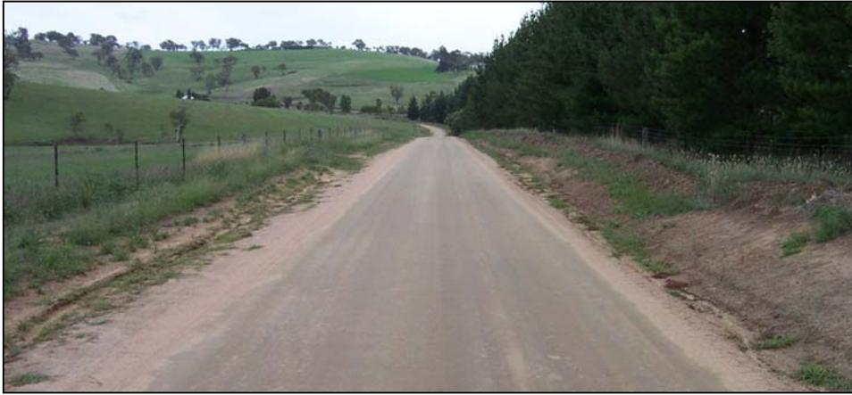
**Figure 2** Unsealed road stabilised with lime to suppress dust generation and provide stiffness to carry heavy traffic loads.
