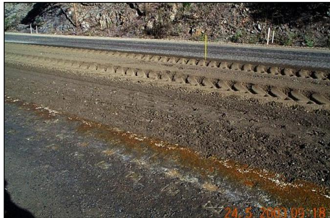
**Figure 9** Leaching of a chemical binder during construction that needs attention.
