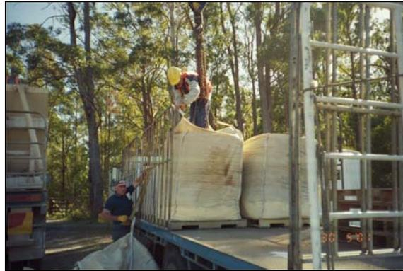
**Figure 7** Bulker bags being prepared for lifting by crane to transfer the binder into a specialist spreader.
