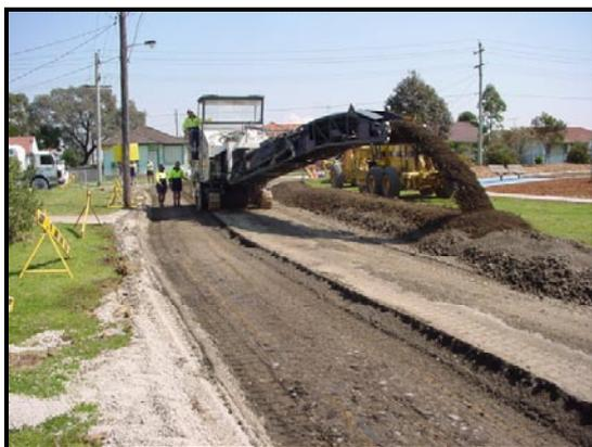
**Figure 2** The subgrade of existing local roads can be stabilised with lime using side casting techniques.
