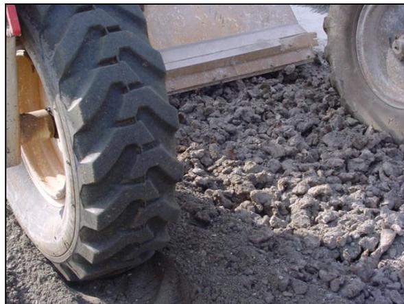
**Figure 7** The first mixing pass with heavy clays will produce material with large pieces of clay.
