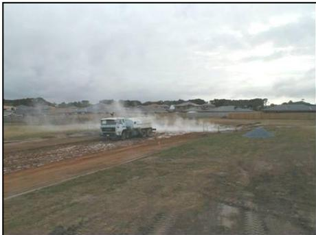
**Figure 6** Slaking of lime produces steam for a short period and appropriate traffic control measures should be considered.
