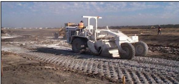
**Figure 1** Lime stabilisation of a weak subgrade for a light trafficked street in a new subdivision.
