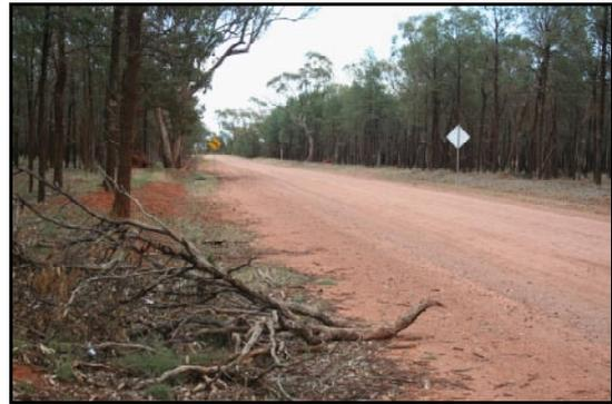
**Figure 3** Unsealed road that was stabilised in 2002 with quicklime.
