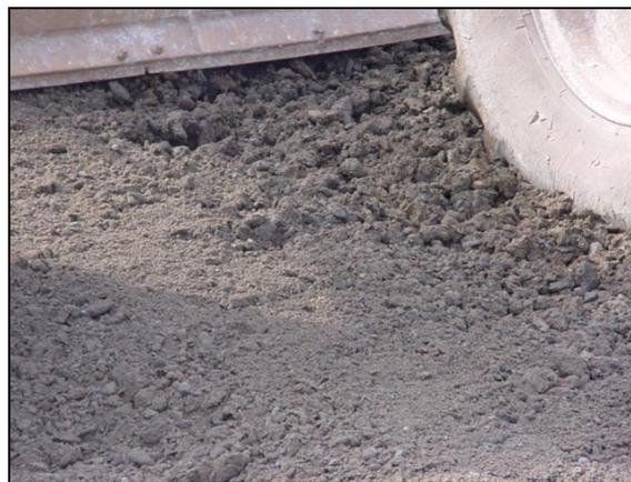
**Figure 8** Subsequent mixing passes with heavy clays will produce finer material suitable for compaction.
