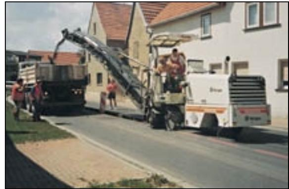
Figure 2 View of a typical profiler.
