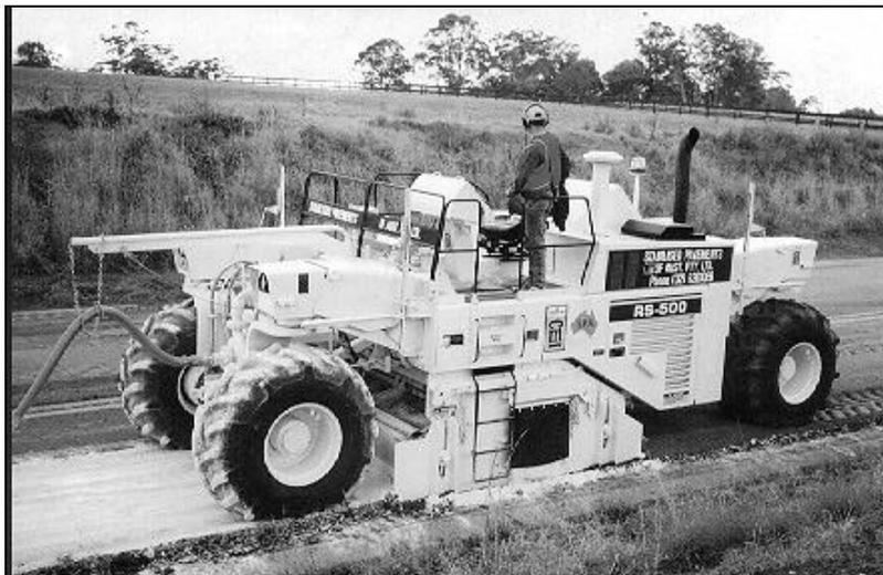
**Figure 4** Lime stabilisation mixing of the Killarney Road project, Warwick.
