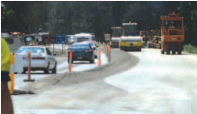
NSW RMS - Farlow's Flat - Plant mixed Foamed Bitumen stabilisation works completed under traffic
