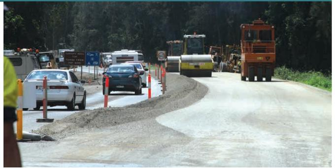
As this is a new research area for RMS, the *Austrad's Guide to Pavement Technology* principles was applied to the project, which was designed as a continuously bound layer, with the expected modes of distress being rutting and/or shoving due to insufficient resistance to pavement deformation and cracking due to fatigue.
