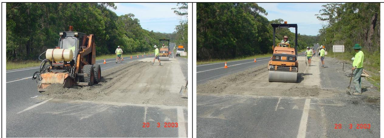
**Figure 3** View of skidsteer and smooth drum roller system for small pavement patch repairs.
