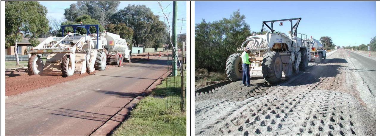
**Figure 2** DPP being used in urban and rural sites using conventional insitu stabilisation equipment.
