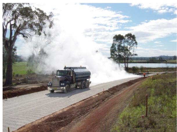
Figure 2 - Slaking of Quicklime in the field
